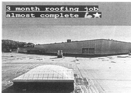
Rye Elementary School roofing / skylight work
