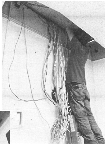
Old Wiring being pruned out
